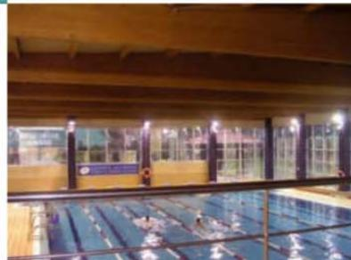
Resistance to corrosive chemical agents makes also timber one of the best material construction choice. For instance, in case of covered swimming pools, due to wet and chlorine environment, timber is the irreplaceable construction material since steel and concrete will be affected by this corrosive atmosphere.
